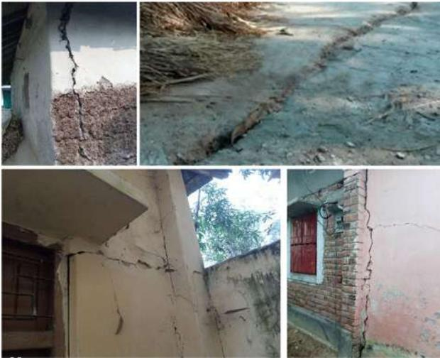
**Fig. 13** Surface cracks and shattered walls found during the field visit in the northern part of the study area
